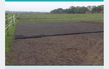
For an all-weather grass surface with excellent mud control, install on a free-draining sub-base, backfill the area with topsoil and then seed or turf for use instead of a sacrifice area. For soil-protection and mudprevention in areas like paddock entrances, extend the paved area by approximately 16 ft into the paddock – maintenance and mowing are unaffected.
